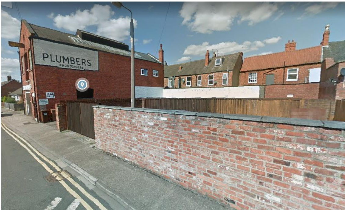
View west towards Princess Street Garage (Google Street View)
