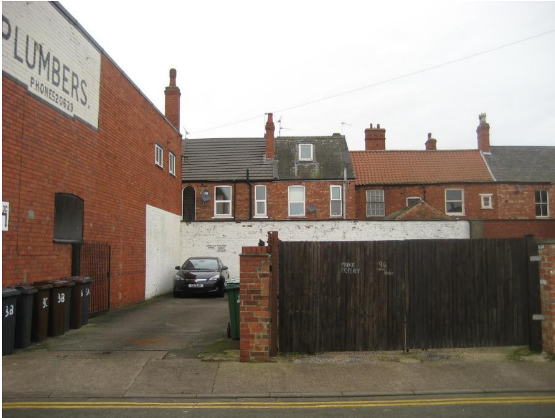
Access to site adjacent to side elevation of Princess Street Garage to the left and north boundary with properties on Foster Street and St. Georges Court in the background.
