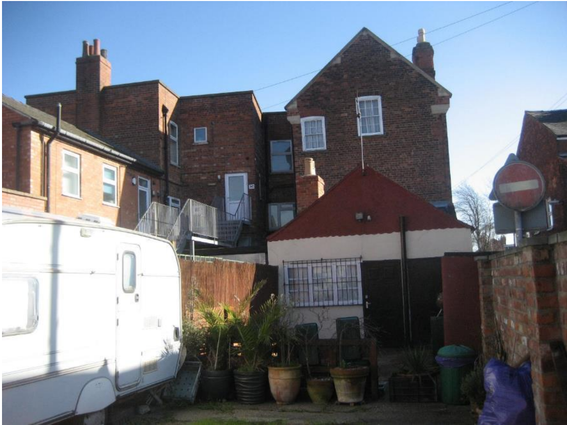
Rear elevation of application property from within the site with High Street properties and 3A-3D Princess Street to the left
